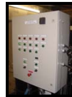
PLC Control Panel
